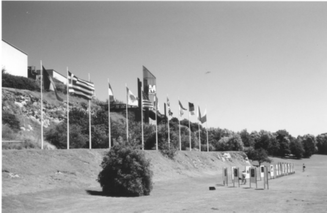
The medieval quarry which forms the garden area at the rear of the museum, as seen from the Canadian Memorial Garden. Part of the new addition is visible at the top left. The displays on the right are a recent addition.
